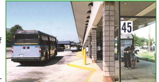
Photo: CCT Marietta Transfer Center
